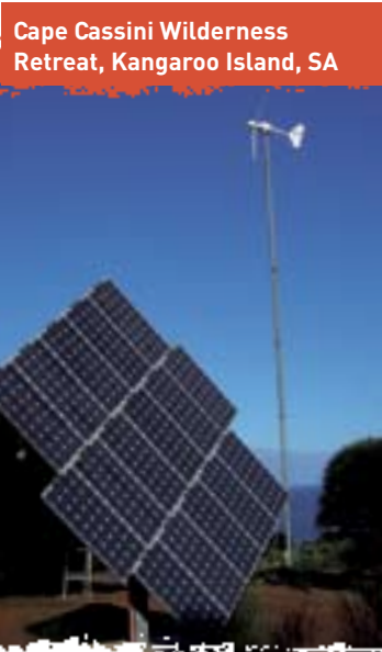
A remote area power supply system, incorporating a tracked solar system, wind turbine and back-up diesel generator, provides all power needs for occupants at Cape Cassini.
