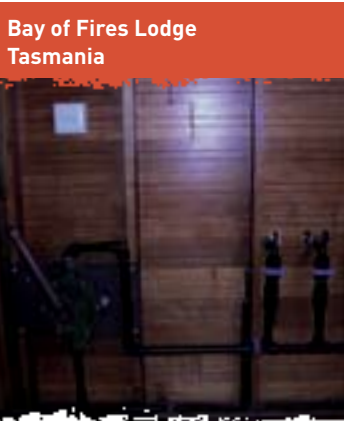
At Bay of Fires Lodge, collected rainwater is adequate to supply all needs. A hands-on approach to handling water (hand pumping of water to header tank before use) and visibility of tanks allows guests to appreciate the amount of available water and how much they are using, encouraging water conservation.
