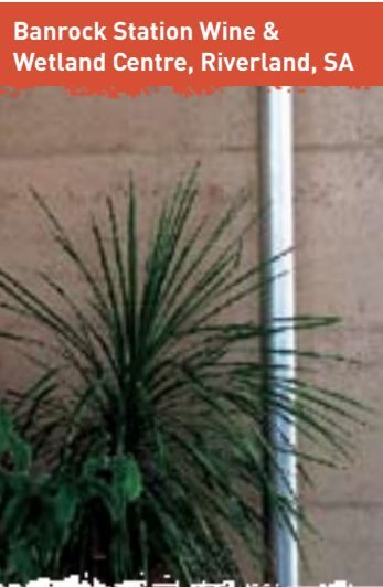
Rammed earth has low embodied energy during construction. Rammed earth has gained popularity as a building material because of its thermal mass properties and aesthetic appeal.
