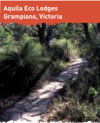
Local stones have been placed loosely to create paved pedestrian pathways and prevent erosion.
